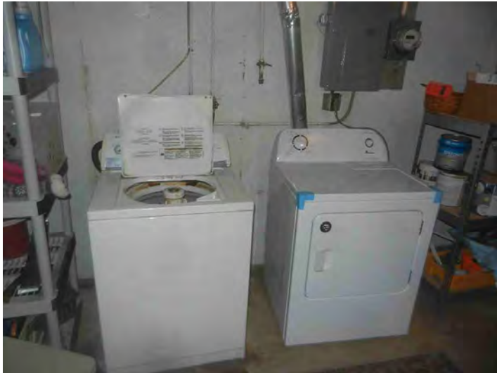
Laundry in basement
